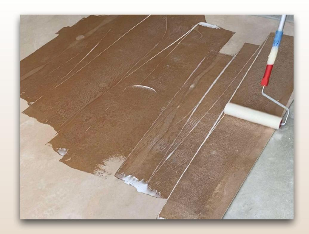
Apply first the primer on the ground base, pouring on it its sand or quartz aggregates, and profile for color geometry. Once fully dry, mix and pour the base on its for a perfect grip.
