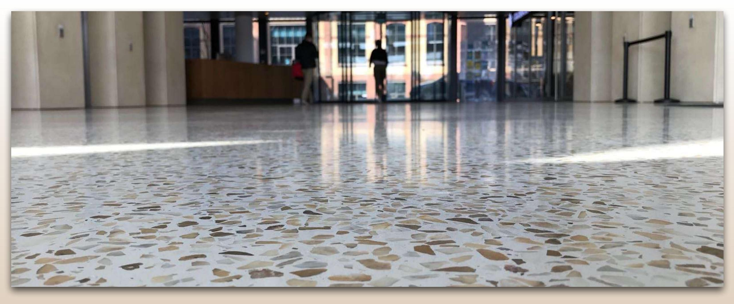
A two components mineral based screed, EPOXY FREE, that can be used to create uniform floors with micro or big aggregates exposure, ground and polished to the desired effect and result, entirely SEAMLESS and no joints!
